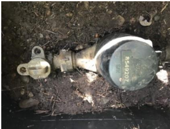
Figure 1. Water shut-off valve, open
